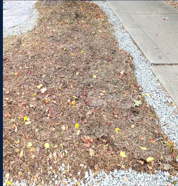
Weed barrier removed & fresh tree mulch & drainage rock perimeter
